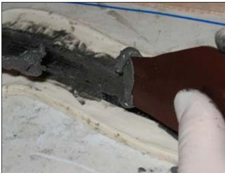
Spreading the micro balloons
