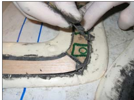
Filling the gap between the balsa and edge...
